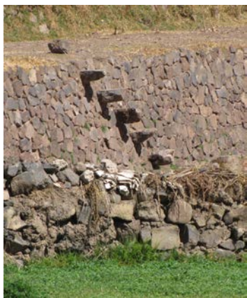
left: Some of the old "stairs" built right into the walls.
